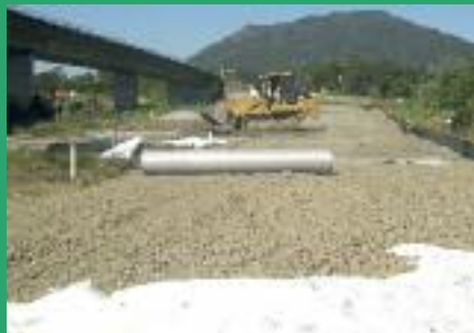
Фиг. 4 Combigrid® unrolled and covered with topsoil
